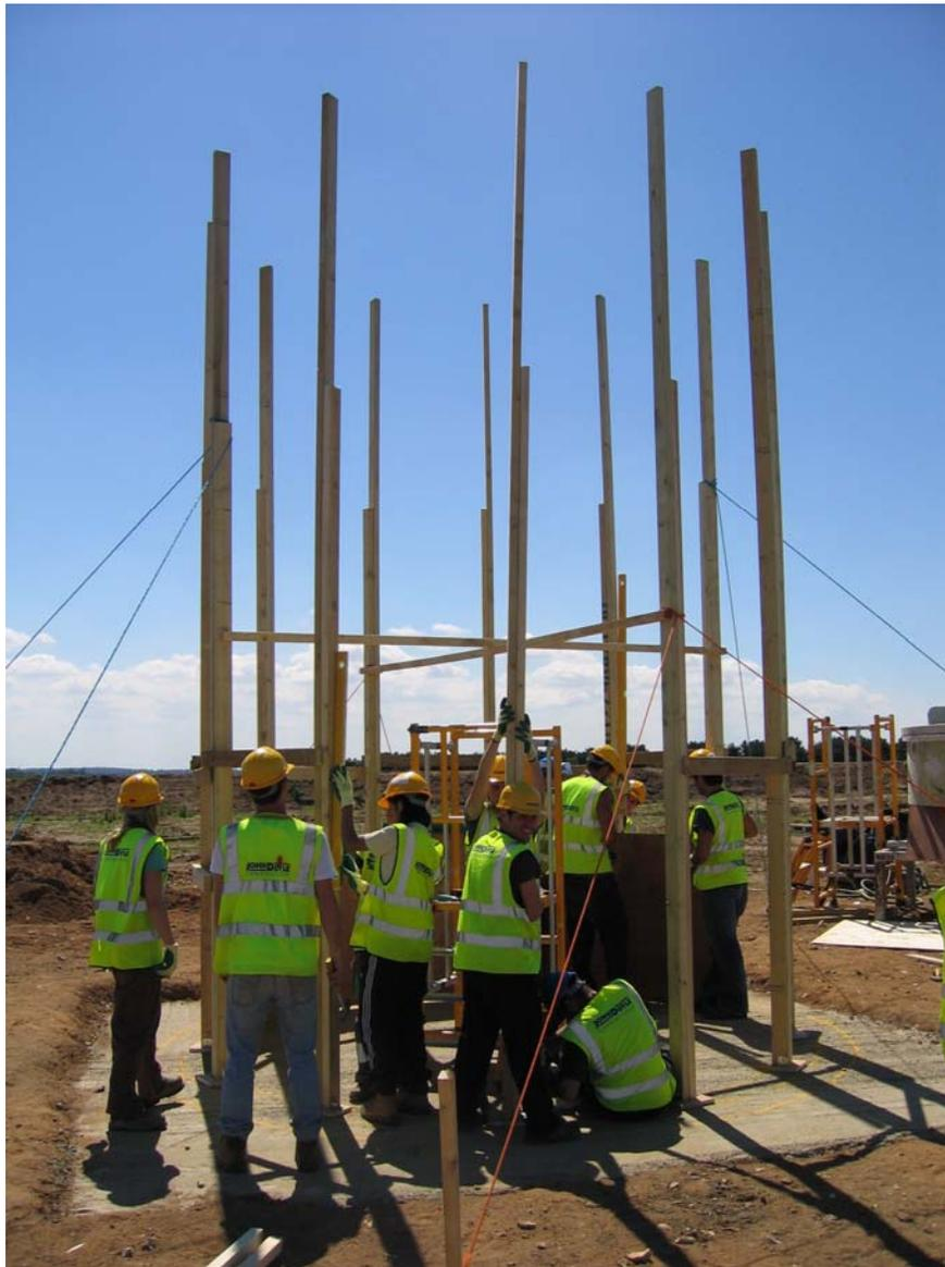
*Guy ropes and horizontal braces used for temporary stability of tower*
