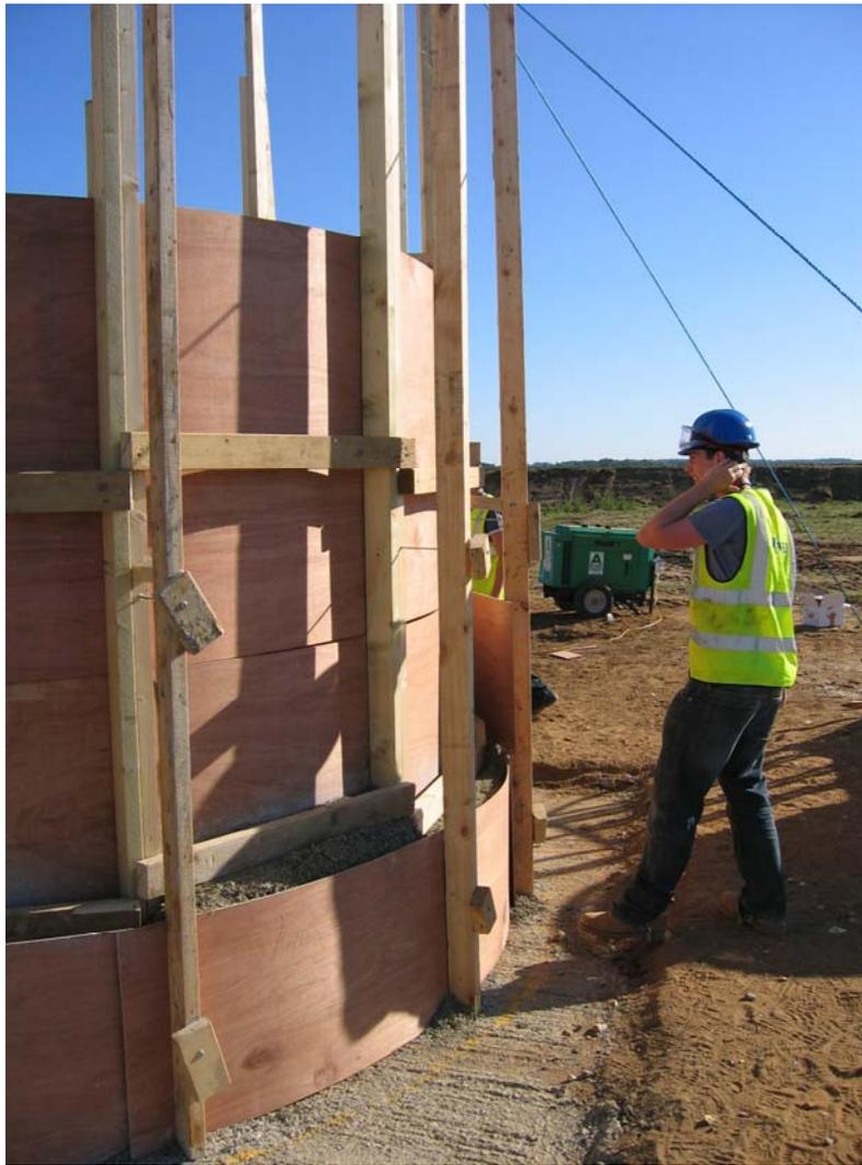
*Outer shutter in 600mm lifts spaced off inner studs using very long screws*
